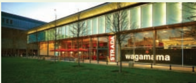
Old Eldon Square – the western side of this key city centre public space has been revitalised by introducing two street level restaurants and a light curtain wall replacing the former brick façade. Further landscaping works will be carried out next year.
