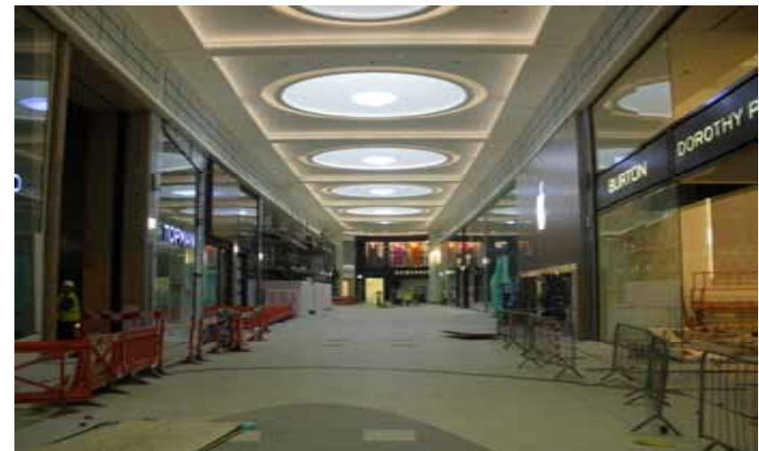
St Andrew's Way during shopfitting
