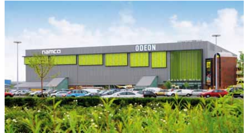
Metrocentre Qube, external view
