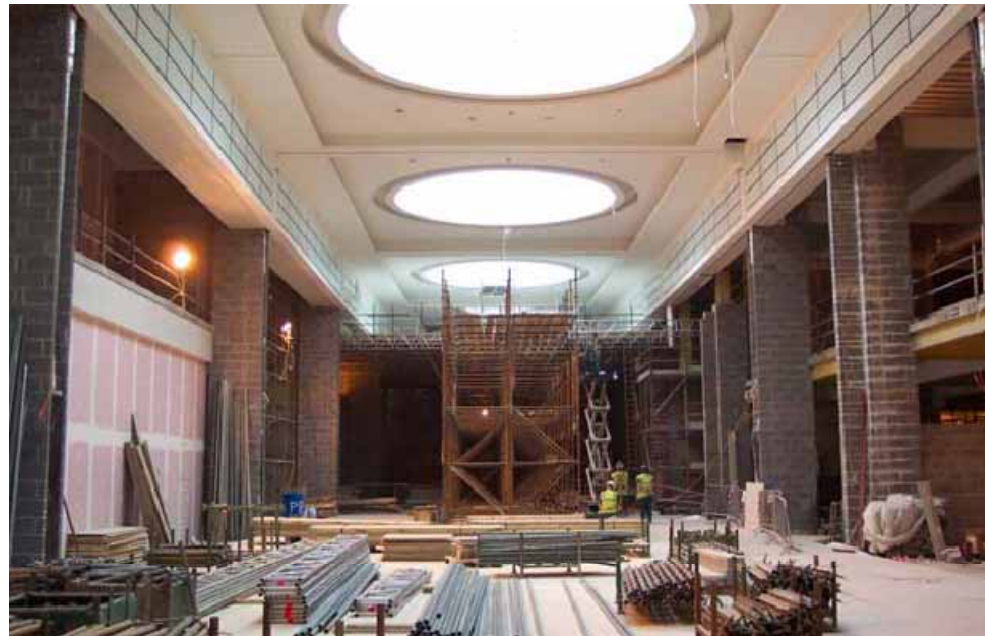
St Andrew's Way during construction
